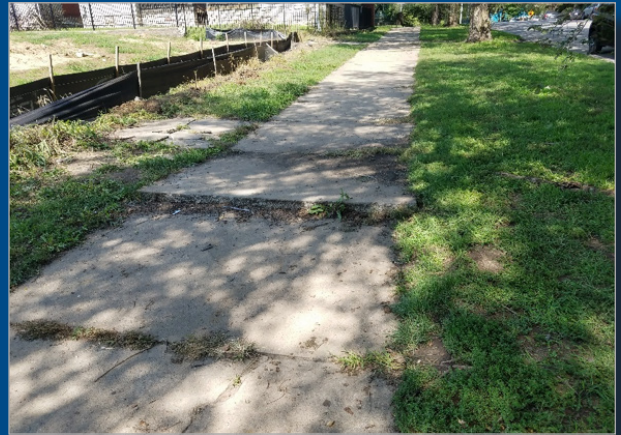
Figure 38: Westside of Maple, Looking North - Spot Treatment Example
